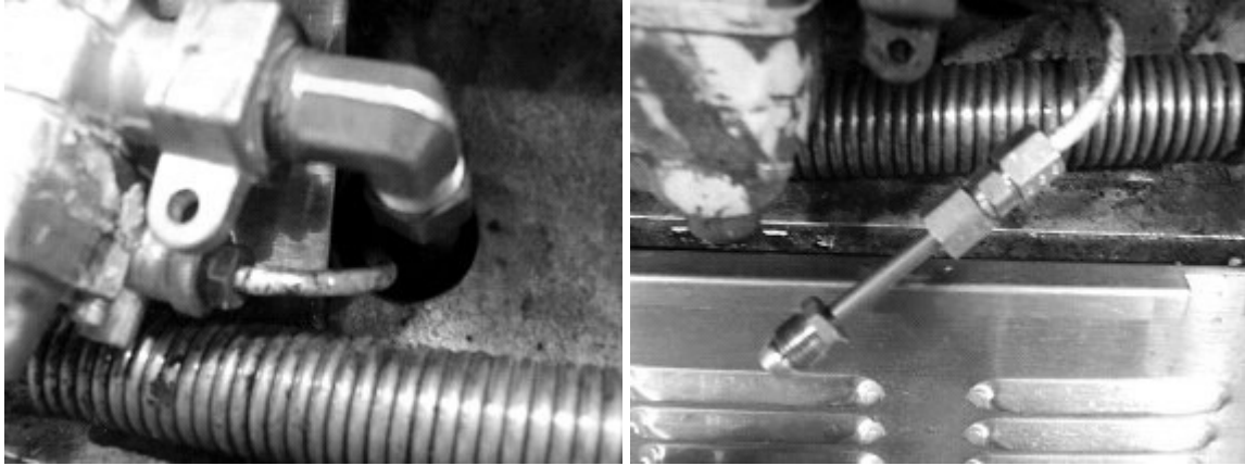
Left: Before extension added Right: After extension added
