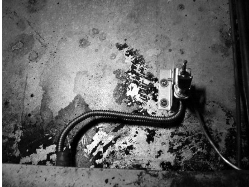
Installed Pilot Assembly. The thermocouple is routed through gas tube opening in the air shield
