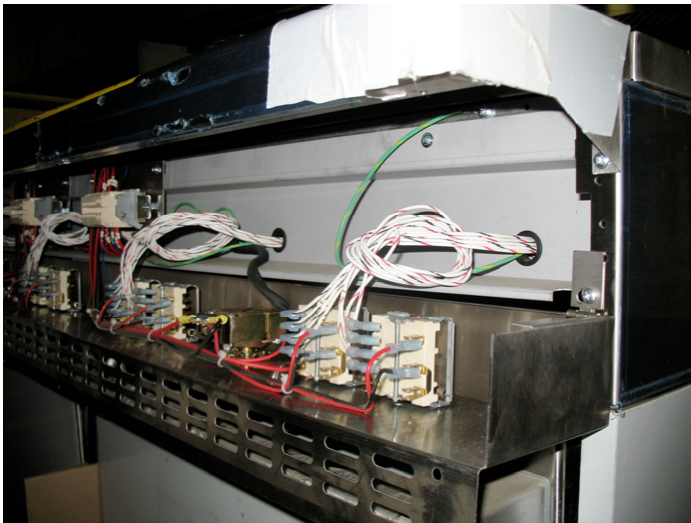
3. Without the screws, the panel will hinge downward.
