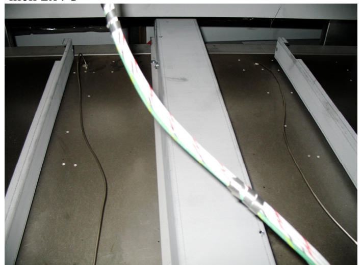
6. The capillary chase is now visible, and the Thermostat may be installed. (Take care not to pinch the capillary when installing)
