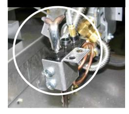
**2.3 Install Field Kit Burner Box**: Engage cut out located at the rear of the burner box over the unit main rear channel and lower the burner box into place.
