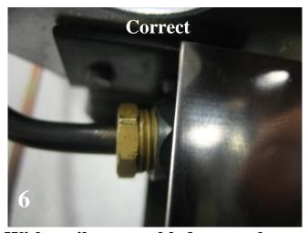
With a pilot assembled correctly approximately 2 threads will be visible.
