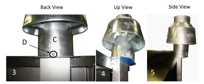
Now install the 6" Direct Vent Bell (C) to the Flu adapter with the single screw (D) as shown in figure 3. The unit is now ready to install the vent pipe according to your local building codes.
