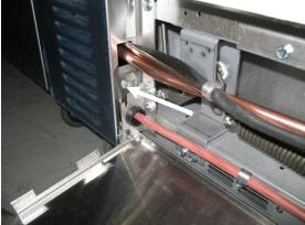
Now remove 2 screws holding the center column panel in place on right side. Left side has a push on pin holding panel, pop panel forward [use caution, the convection oven switch is mounted to this panel].
