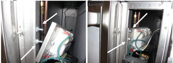
\*Before beginning this step: make sure that the Module is wired correctly (as per appendix A)\* Once ignition module is mounted on the provided bracket, open the Control column and insert two 10-24 bolts through the frame and tighten down with nuts as shown. Place ignition module assembly onto bolts through the holes on the bracket and install two more 10-24 nuts securely.
