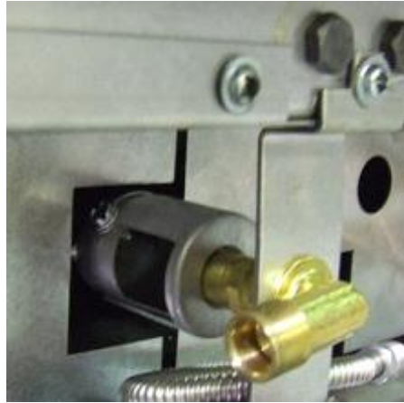
Orifice inserted straight into burner opening
