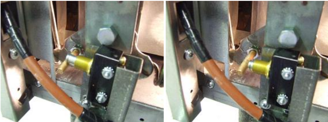
Left: INCORRECT. Button is not depressed when bracket is screwed on Right: Correct installation with depressed button.
