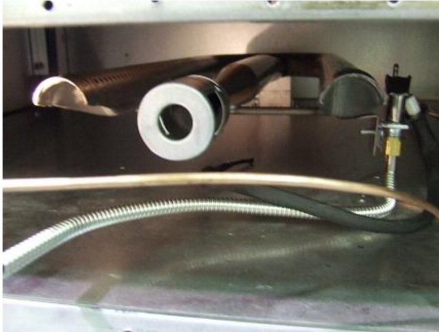
New burner and pilot assembly installed
