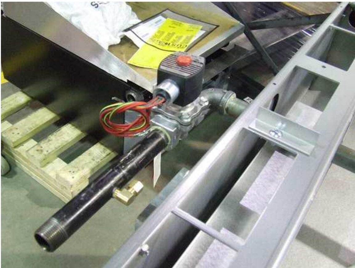
Installation of Solenoid Valve and Piping
