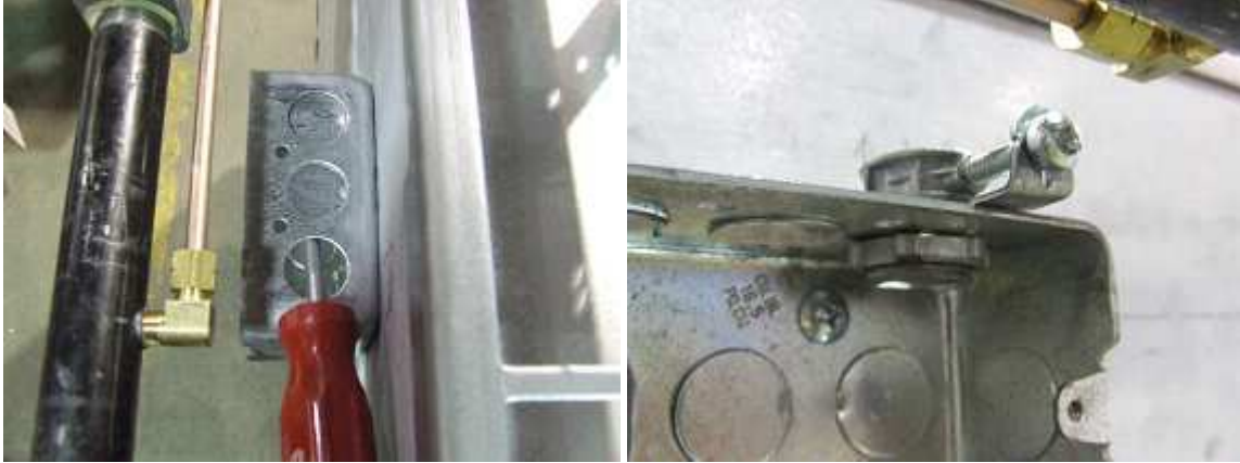
Left: Removal of Circular Tab Right: Installation of Unmodified BX Connector
