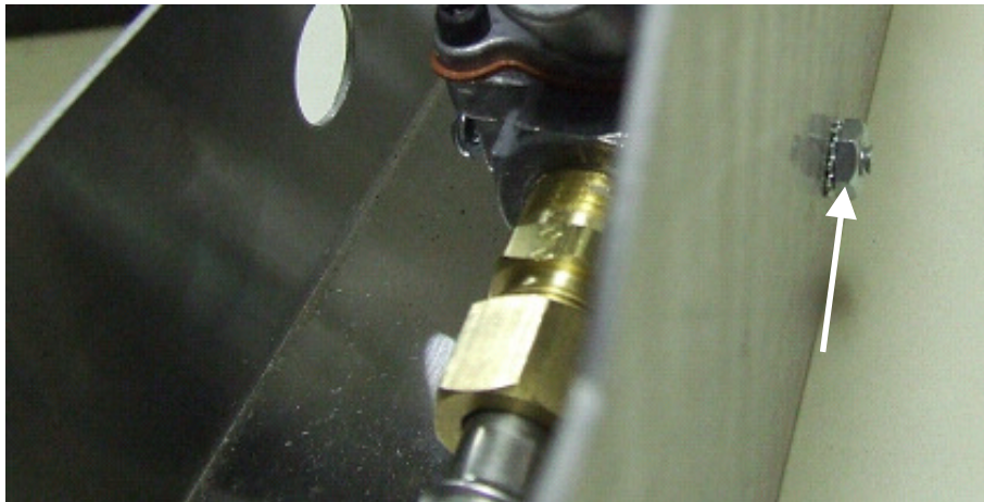
Nut holding bolt in place on back of bracket
