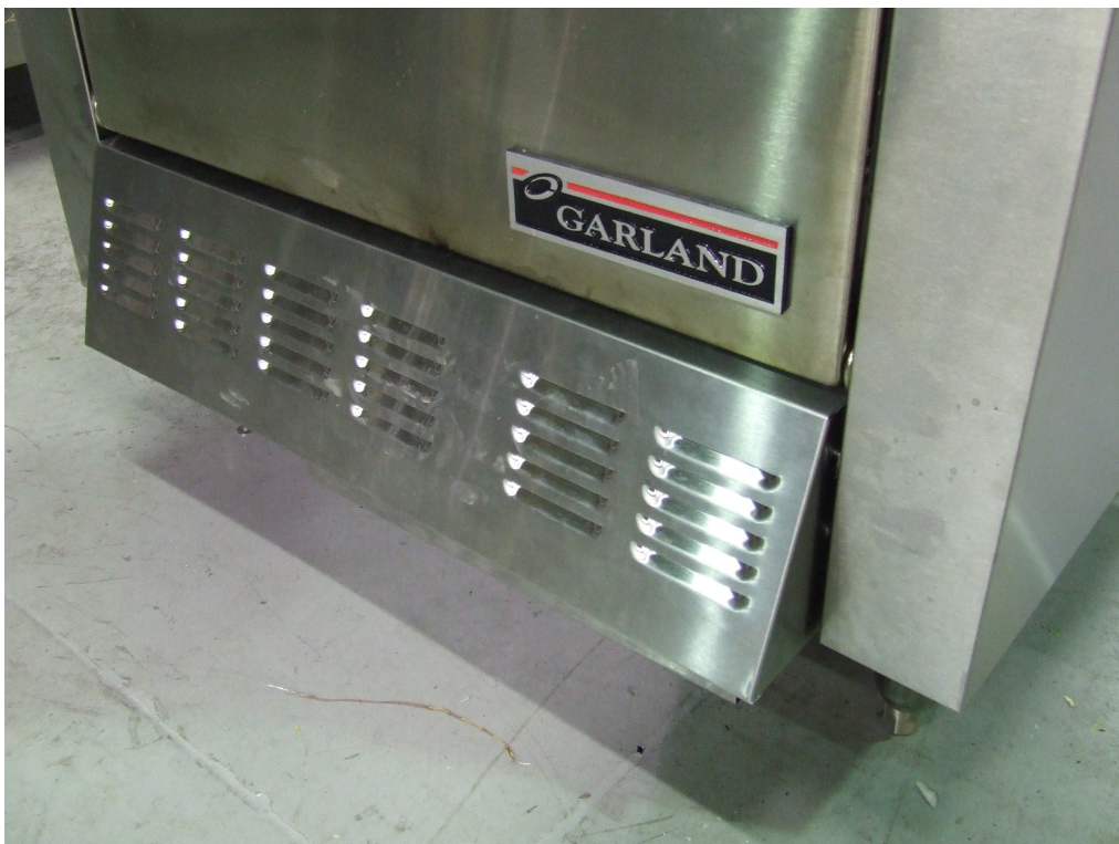
Installation Complete – Kick Plate On
