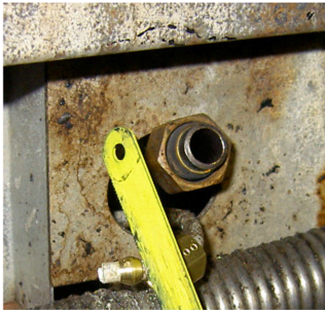
Use of hacksaw blade to remove tip of pilot gas line
