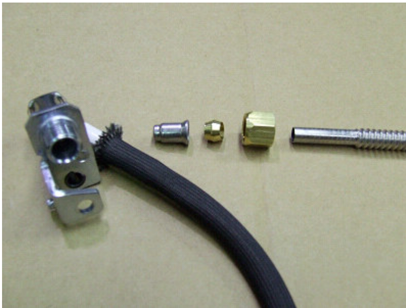
Nut on new pilot assembly unscrewed, revealing orifice and ferrule.
