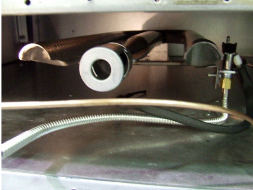
New burner and pilot assembly installed
